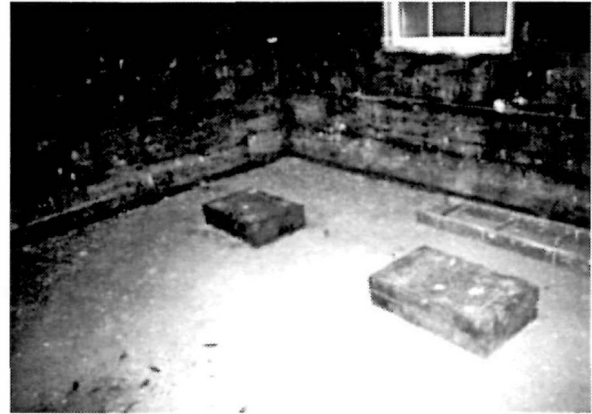
Figure 31 Interior view looking northeast inside of the Fog Signal Building, 1994.
