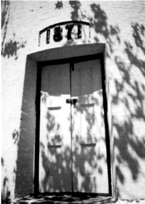
Figure 41 Detail view of the pair of doors at the base entrance into the Tower, 1994.
