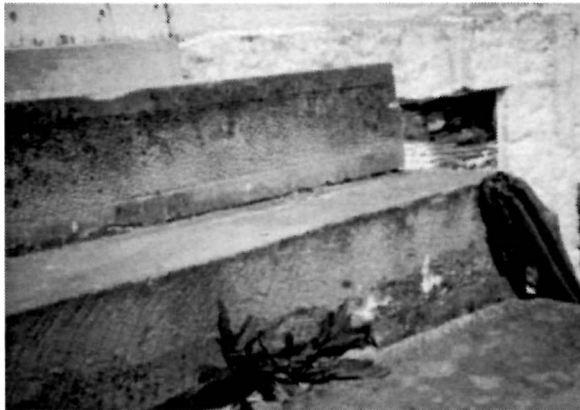
Figure 30 Detail view of the exterior concrete steps leading to the main entrance into the Keeper's Dwelling along the south elevation, 1994. The face of both the top riser and the door sill have an elaborate tooled pattern, while the face of the risers below are less ornate.
