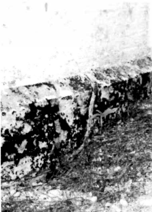
Figure 43 Detail view of the copper grounding cable (part of the lightning protection system) extending out from interior base of the Tower, 1994.
