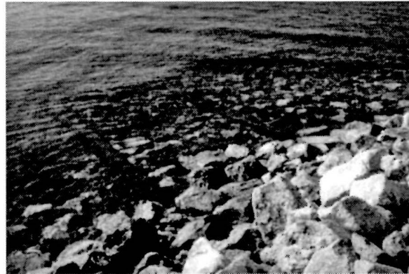
Figure 10 View of the timber cribbing in front of the Fog Signal Building, 1995.
