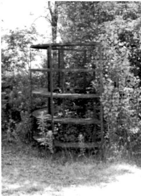
Figure 80 View of the rusted metal shelving previously located inside the Metal Oil House, 1994.
