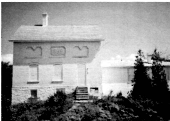
Figure 23 View of the south elevation of the Keeper's Dwelling, 1994. Note the decorative brick recesses at the second floor, and the raised brick "eyebrows" above the door and window openings.
