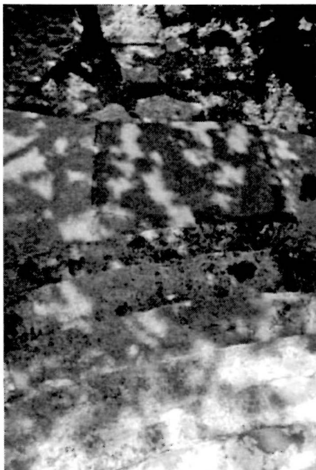
Figure 21 View of the bluestone slab and steps at the Tower, 1995.
