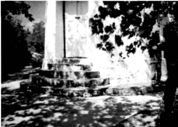
Figure 40 Detail view of the stone steps at the base of the Tower, 1994.
