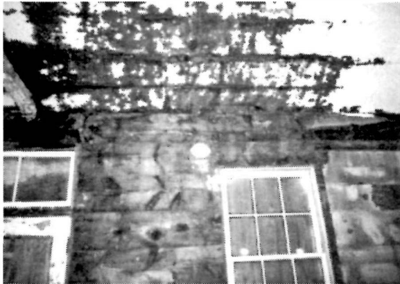
Figure 70 View of the south wall of the Machinery Room in the Fog Signal Building, 1995. Note the circular opening just above the window.
