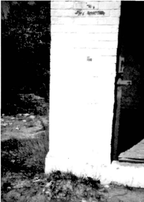
Figure 76 Detail view of the south corner of the east elevation of the Brick Oil House, 1994. Note the parging, which was tooled to resemble brickwork and is falling off.
