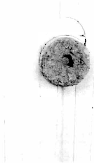
Figure 19 Detail view of the concrete “plug” in the former stovepipe opening at the workroom of the Tower, 1994. There is also another circular marking in the wood wainscot, suggesting that the opening was relocated.
