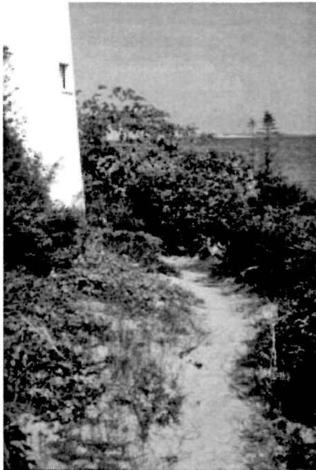
Figure 20 View of the sand drifts over the sidewalk south of the Keeper's Dwelling, 1995.
