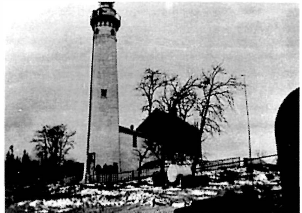
Figure 20 View looking southwest toward the South Manitou Island Light Station, circa the late 1930s. Note the air tanks and air lines which were part of the air diaphone system.
