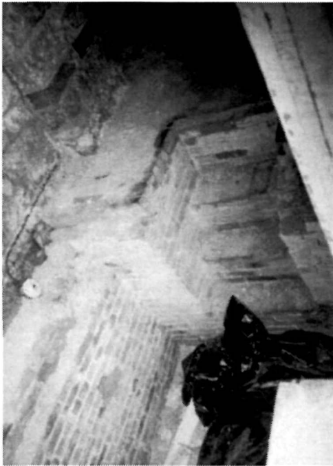
Figure 52 View looking down into the subcellar (Room B-03) of the Keeper's Dwelling, from the stair, 1994. Note the steep brick-lined steps leading down into the subcellar, and the exposed conduit of a former light fixture.
