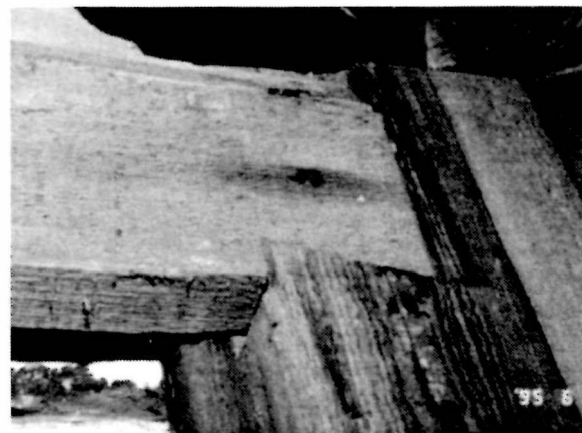
Figure 22 View of the heavy timber joinery at the original Tower, 1995.
