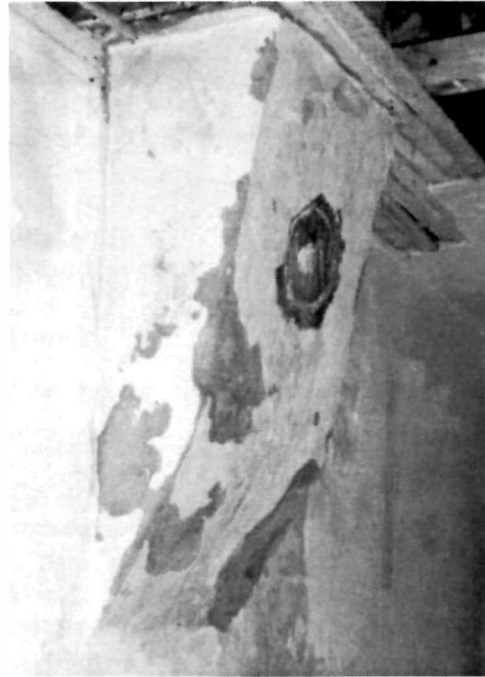
Figure 48 Interior view of the chimney in the Passageway, which is corbelled in from the wall approximately 5'-0" above the floor, 1994.
