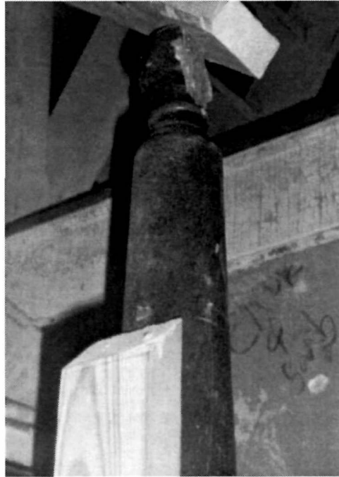
Figure 61 Detail view of the intermediate newel post, the only remaining element of the balustrade at the stair in the northwest corner of Room 101 of the Keeper's Dwelling, 1994.
