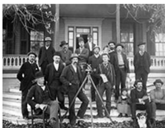
Erastus A. Williams, U.S. Surveyor General, with survey crew, circa 1892, Bismarck, ND. Note the survey transit and chains draped over the shoulders and held by the two chain men. E.A. Williams, a prominent member of the state legislature from 1872 - 1916, served as U.S. Surveyor General from 1890 until 1907. SAHRL E0048
