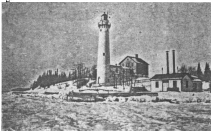
Lighthouse and fog signal – South Manitou during winter 1917 with ice on the lake and snow on the ground, also the two stacks on the boiler room to make steam for whistle during fog and snow storms, also wood in right corner for boilers.
