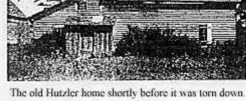
The old Hutzler home shortly before it was torn down.
