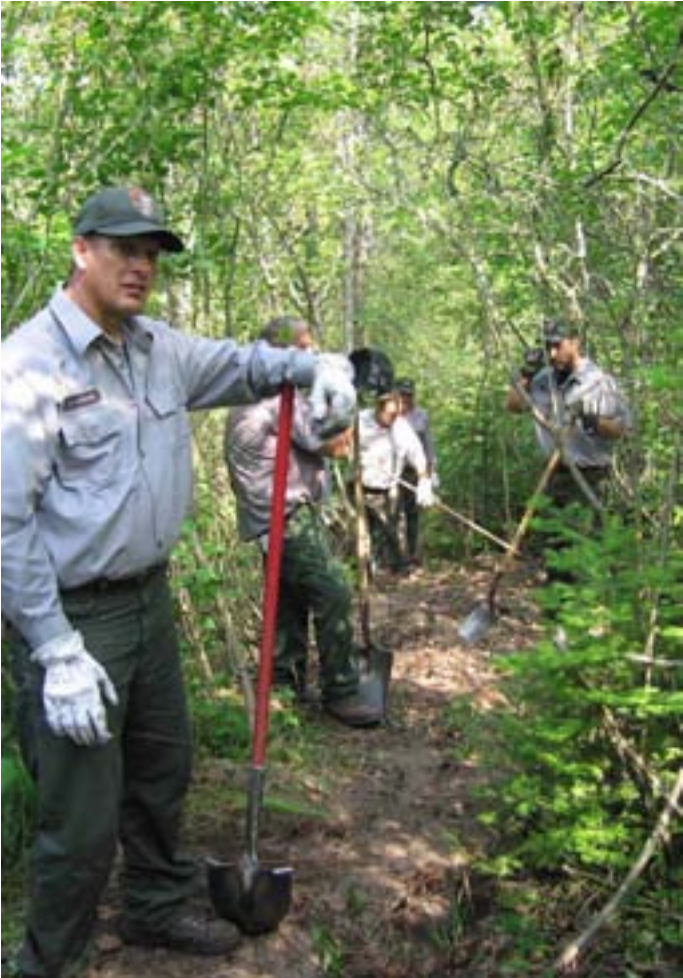
Rangers clear path and lay new underground electrical cable.
