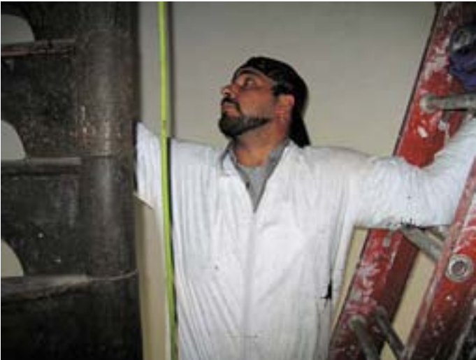
Earl jr - NPS maintenance crew stabilizes and repaints tower interior.
