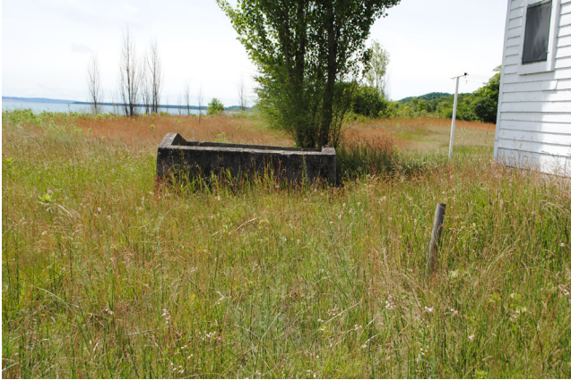
Figure 3-35. Flammable Materials Shed (source: Mundus Bishop, 2024).
