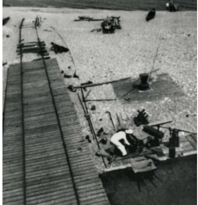
Figure 3-43. View from the roof of Lifeboat Station to the Launchway, Capstan, and Fire Pump, 1926 to 1928 (source: Sleeping Bear Dunes National Lakeshore).
