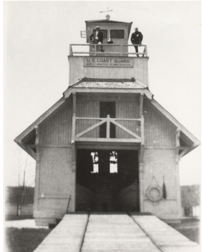
Figure 2-23. Lifeboat Station, taken between 1925 and 1927 (source: Leelanau Historical Society).
