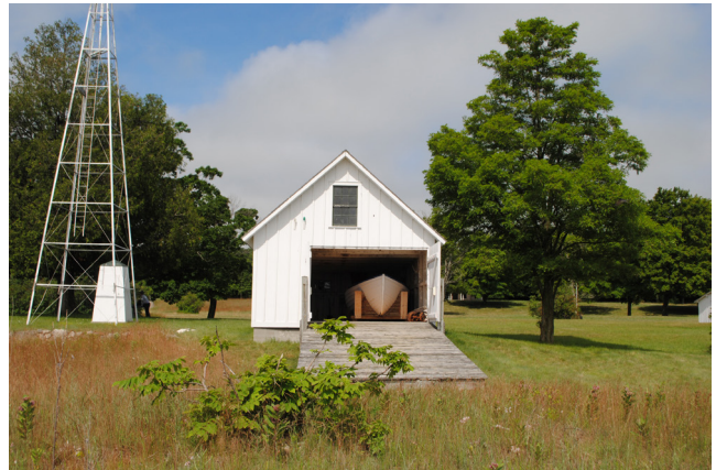
Figure 3-27. Volunteer Rescue Station, Flag Locker, and Storm Signal Tower (source: Mundus Bishop, 2024).
