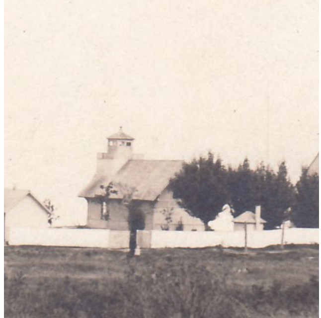
Figure 3-50. Non-extant white picket fence with gates defining perimeter of station (source: Sleeping Bear Dunes National Lakeshore).
