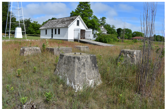
Figure 3-28. Lookout Tower Abutments (source: Mundus Bishop, 2024).
