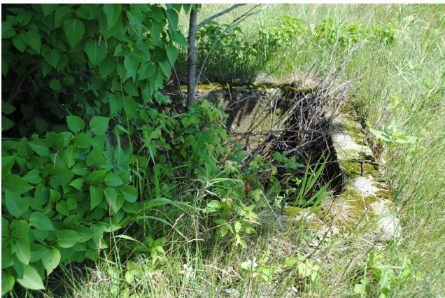
Figure 3-30. Fire Pump Well Foundation (source: Mundus Bishop, 2024).
