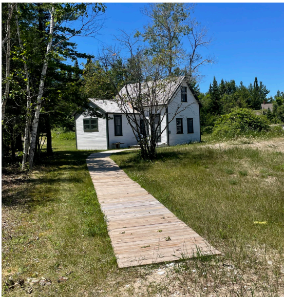
Figure 3-27. Boardwalk access to the Hutzler House (source: Mundus Bishop, 2024).
