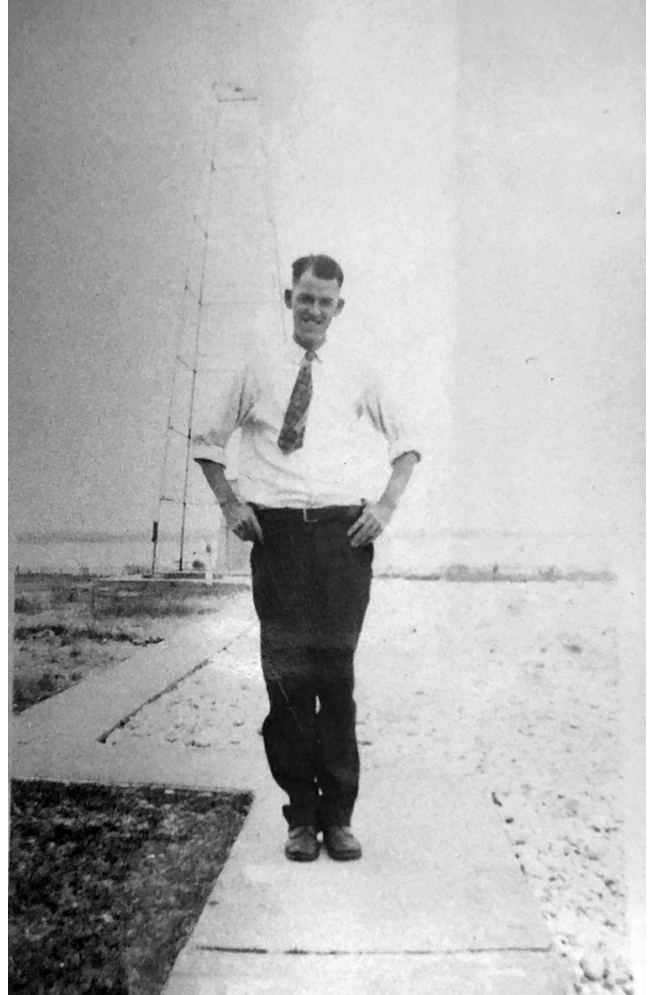
Figure 2-26. Gerry Crowner on concrete walks leading to Storm Signal Tower and Flag Locker, c. 1926-28 (source: National Visual Inventory Cards, Sleeping Bear Dunes National Lakeshore).
