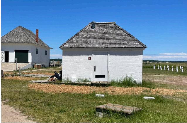
Figure 3-63. Flammable Storage Shed (source: Mundus Bishop, 2024).
