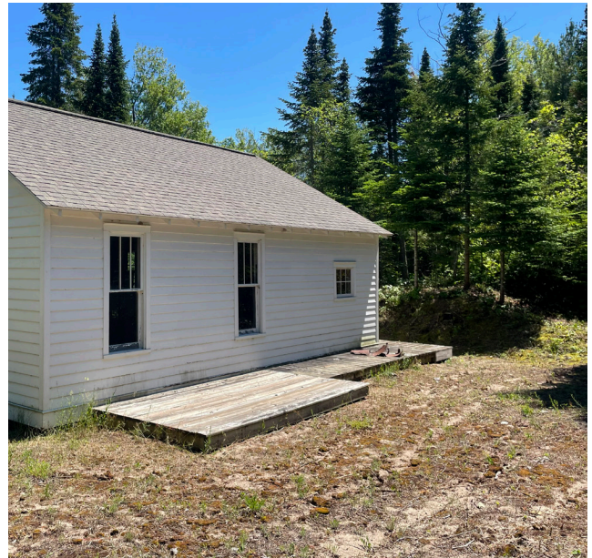
Figure 3-25. Berm south of the Edwin and lola Tobin House (source: Mundus Bishop, 2024).
