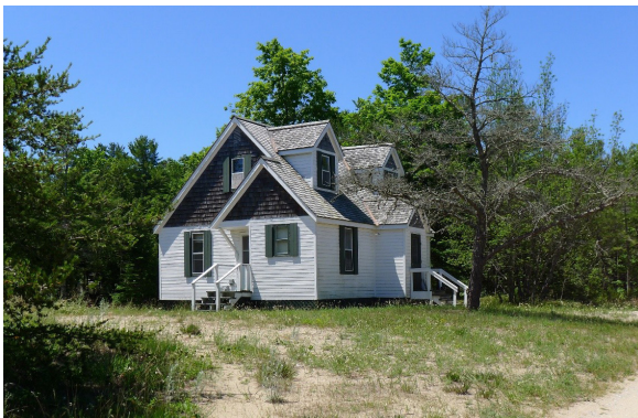
Figure 3-37. The Keeler House (source: Clerestory Preservation, 2024).
