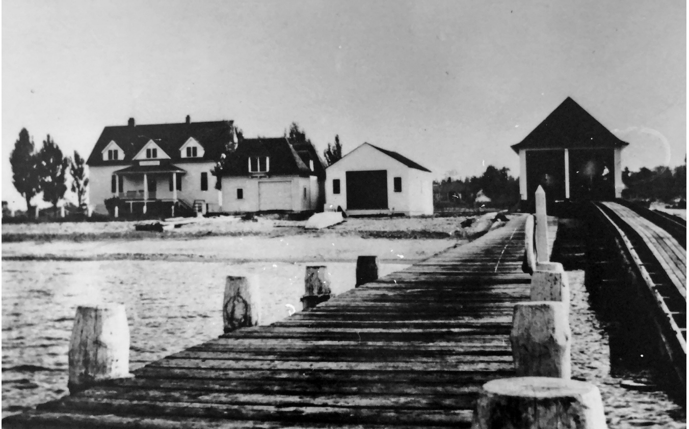
Figure 2-34. Launchway set on wooden piles with two tracks for lifeboats and pile bent dock built in 1932 (source: National Visual Inventory Cards, Sleeping Bear Dunes National Lakeshore).
