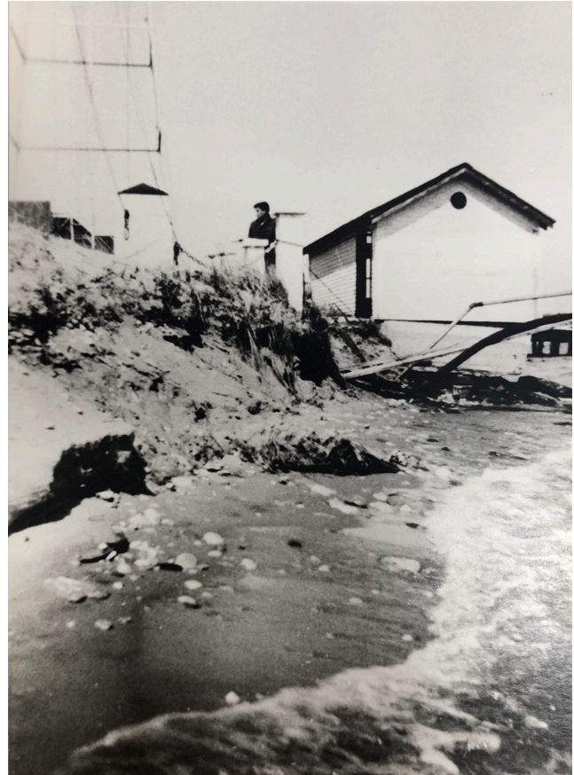
Figure 2-40. Erosion at shoreline, winter 1946. Pumphouse and Storm Signal Tower and Flag Locker are in the background (source: National Visual Inventory Cards, Sleeping Bear Dunes National Lakeshore).
