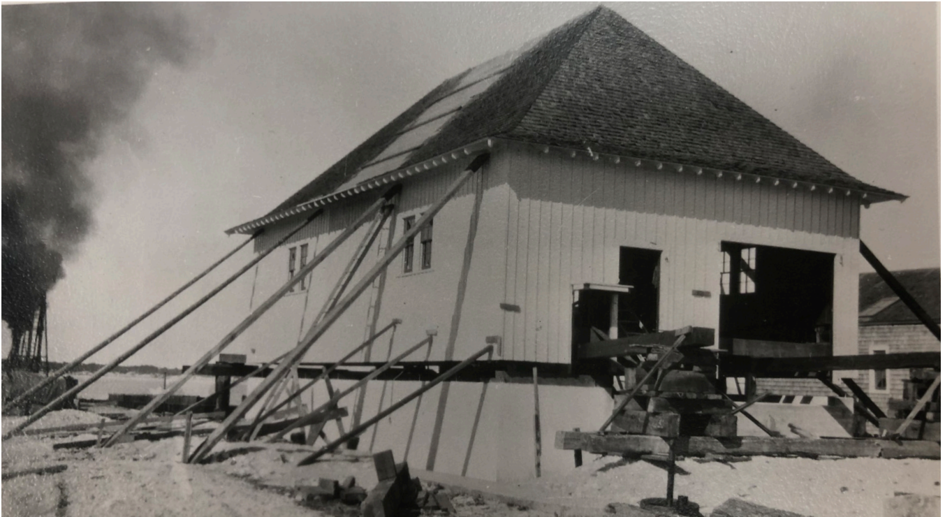
Figure 2-20. The raising of the Boathouse #2, 1916 (source: National Visual Inventory Cards, Sleeping Bear Dunes National Lakeshore).
