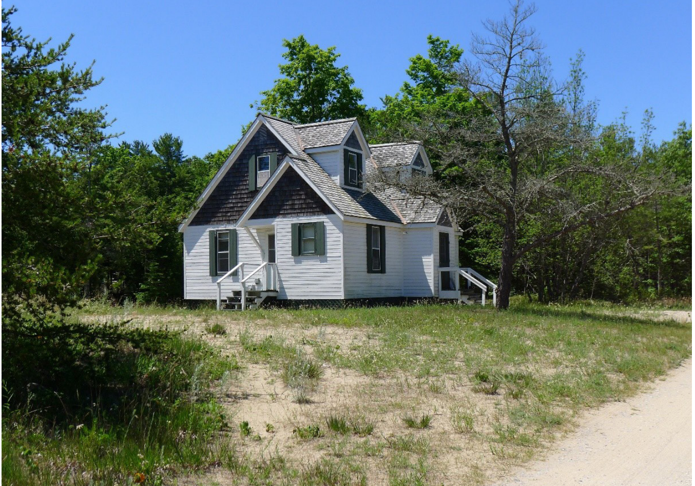
Figure 3-80. Keeler House (source: Clerestory Preservation, 2024).
